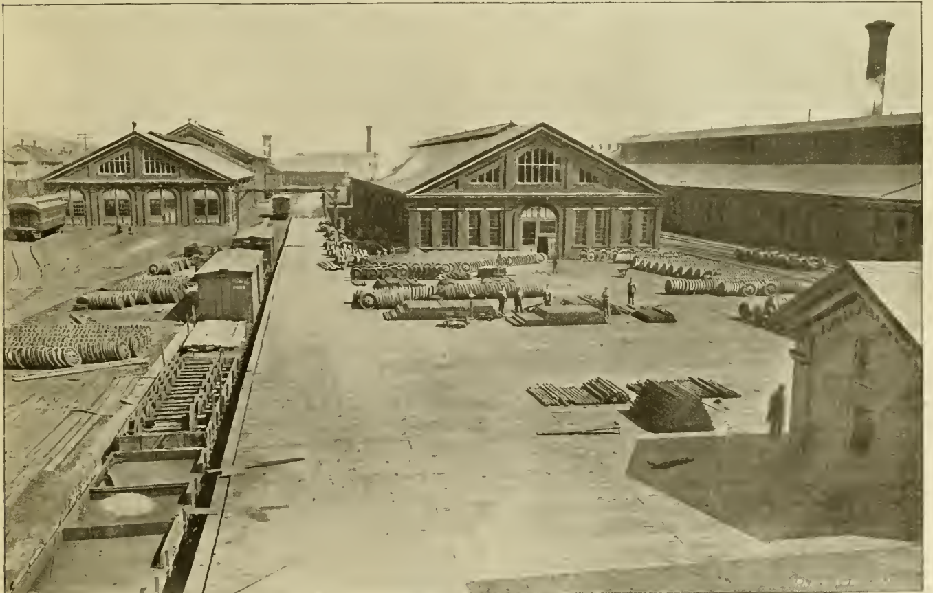
Car Shops of the Pennsylvania Railroad Altoona Pa.
